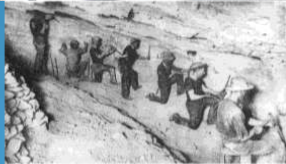
Single jockers working in a mine in the Gouldenough Mine, circa 1890 Marie Devere Collection
