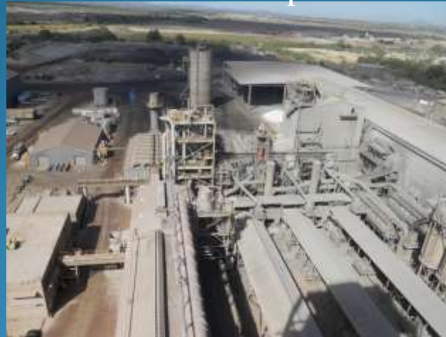
Rillito Cement plant
